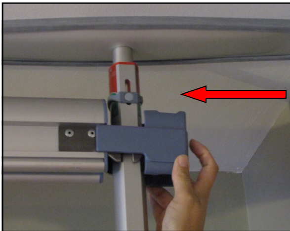
Step 14a: Attach the track end cap as shown above.
