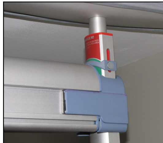
Step 14b: Install the other end cap.
