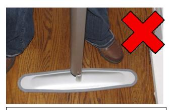
NOTE: **Never install Top Foot** at the Bottom section of Post
