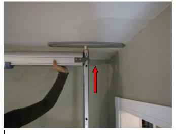
To Unhook the track assembly, lift the track up from one post end.
